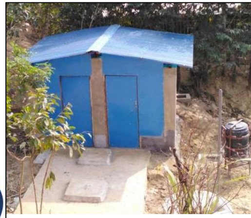
Pit latrines, Septic tanks
